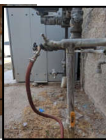
Potable: 2nd source of shutoff
