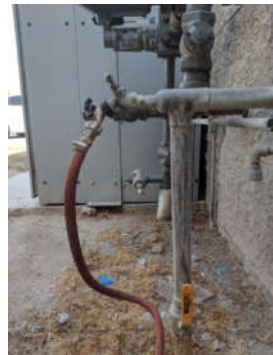
Potable: 2nd source of shutoff
